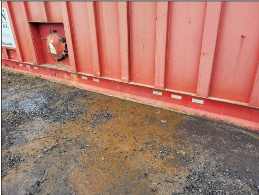
Photograph 2 (March 27, 2023). Frac tank showing evidence of leakage (rust coloured staining on ground).
