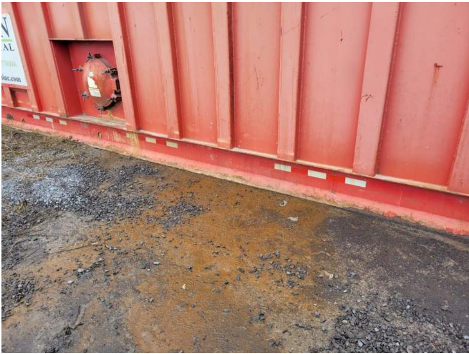
Photo 1: Soil staining resulting from leachate released from leaking frac tank (March 27, 2023)
