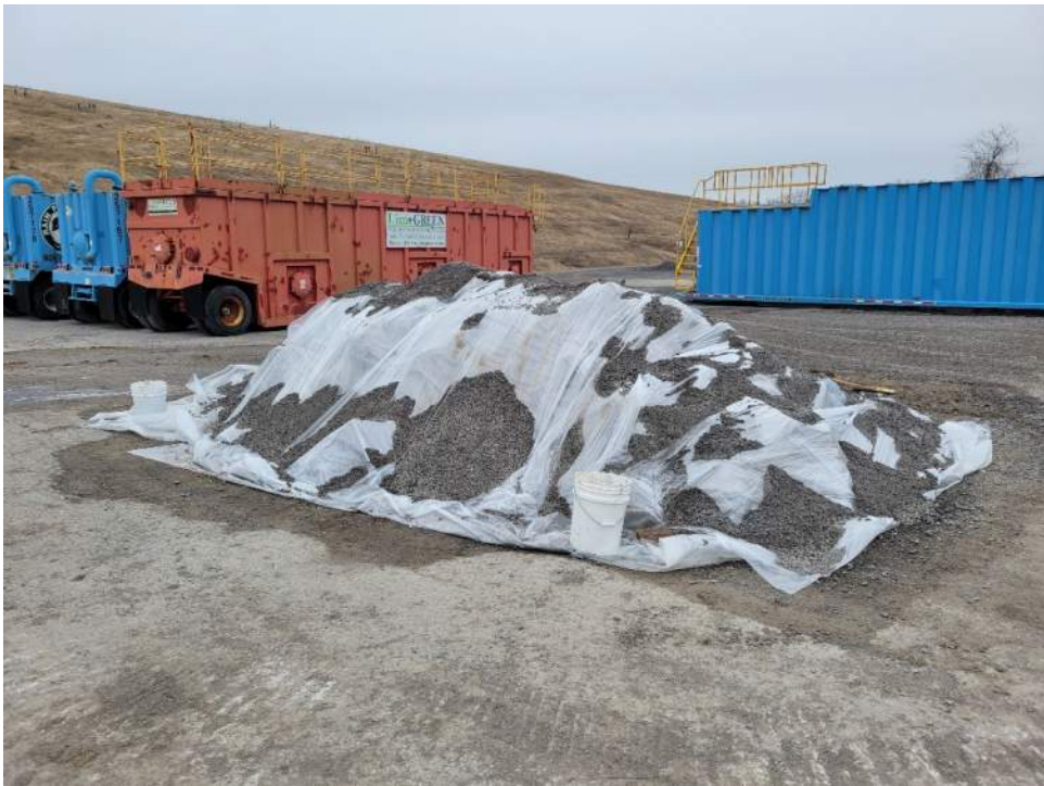
Photo 3: Stockpiled impacted soil (March 30, 2023)
