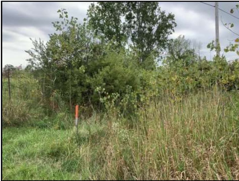
Photo 10: View facing southwest of the Stormwater Pond 3 spillway channel outlet to the north ditch along Beechwood Road. The outlet is becoming obscured with thick vegetation.
