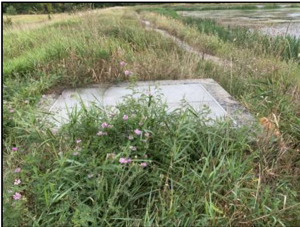
Photo 24: View facing east of the northwest structure at the leachate holding lagoon. “Confined Space” signage was not observed.
