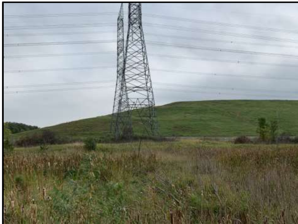
Photo 34: View facing south of the northeast landfill mound. Brown patches are visible at locations of former seep repairs.
