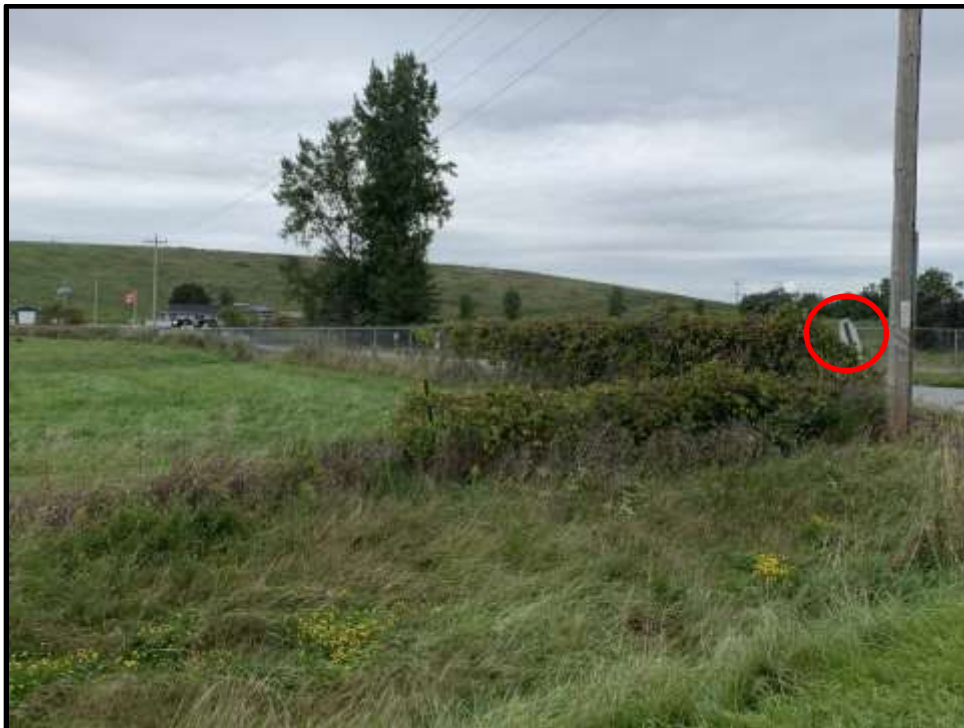
Photo 6: View facing southwest of the Stop sign at the landfill entrance. The Stop sign is leaning away from the traffic sight line and thick vegetation is obscuring additional signage on the fence.
