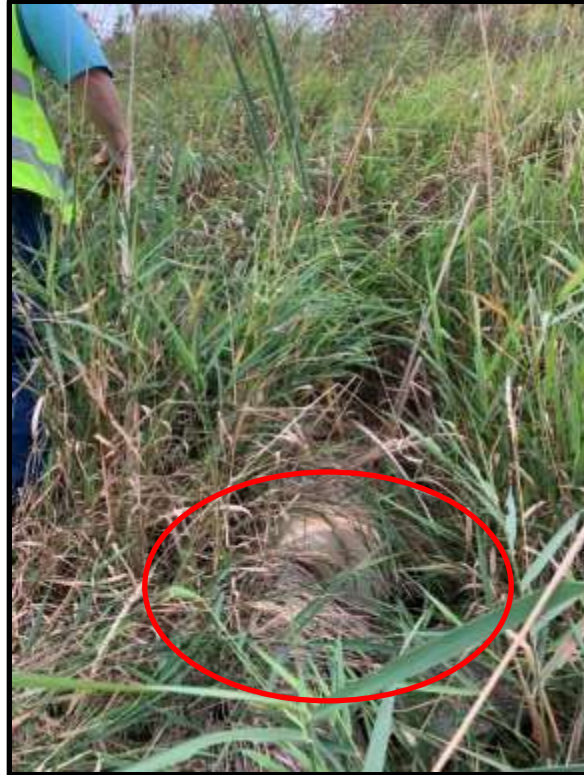
Photo 33: View of the outlet pipe from the drop inlet pipe structure at Stormwater Pond 1. A cap is present on the outlet pipe.
