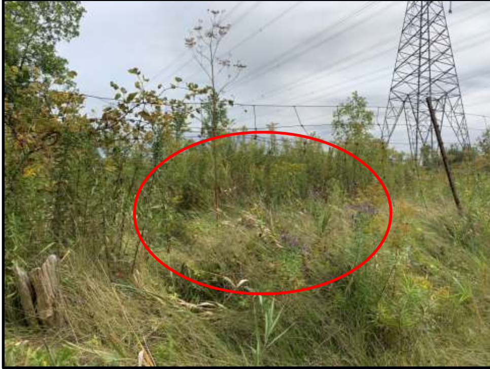
Photo 9: View facing east of a hole in the Paige wire fence along County Road 10, east of hydro tower ID X527B and west of monitoring wells 82-1 and 82-2.
