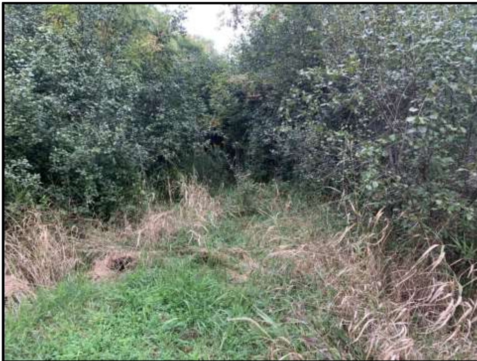
Photo 18: View facing east of the northeast path around Stormwater Pond 2. Vegetation has obscured the path, restricting access.
