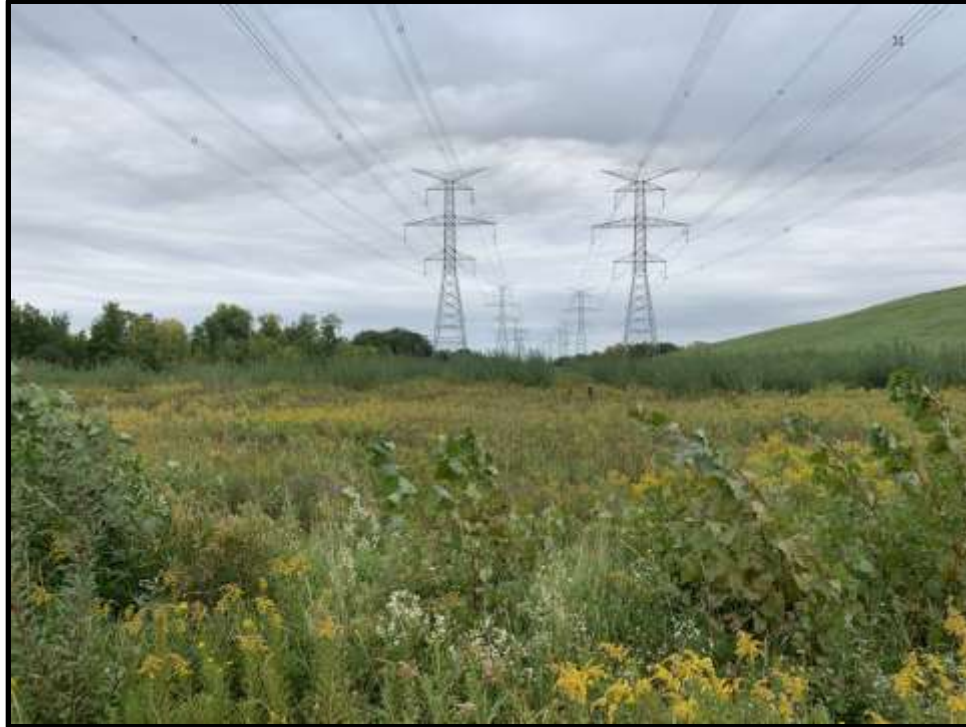
Photo 15: View facing east of the phytoremediation system. Vegetation was pruned by Hydro One in spring 2021.
