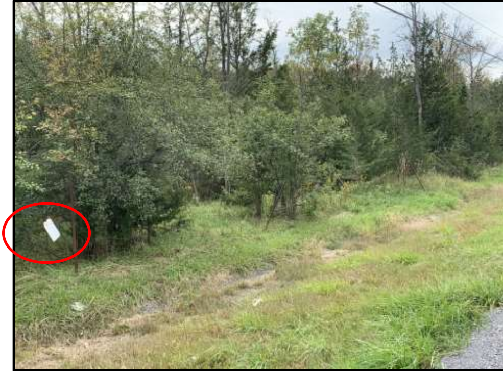
Photo 7: View facing southwest of a section of the north perimeter fence along Selby Road, east of the former Wildlife Habitat house. Fence posts in the area are leaning, the paige wire fence is down, and the “No Trespassing” sign (circled) is not visible.
