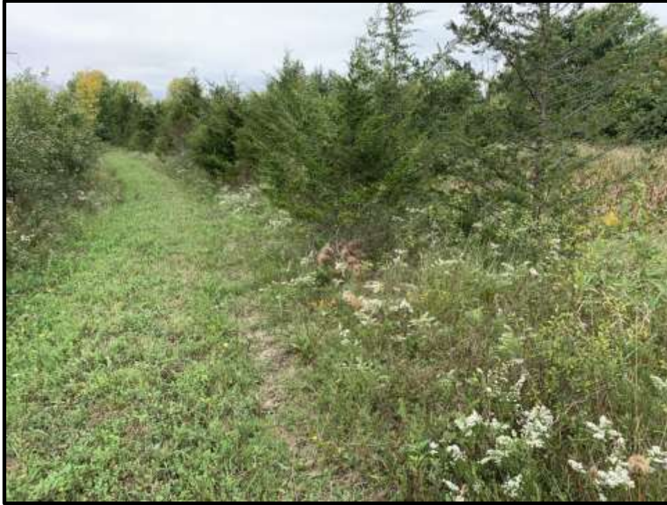
Photo 17: View facing west of the path along the south side of Stormwater Pond 2. Large trees are present on the interior of the pond.
