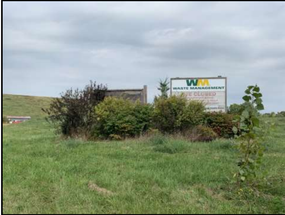
Photo 5: View facing northeast of the signage east of the landfill entrance. The sign is becoming obscured by vegetation, which affects visibility of the contact information.
